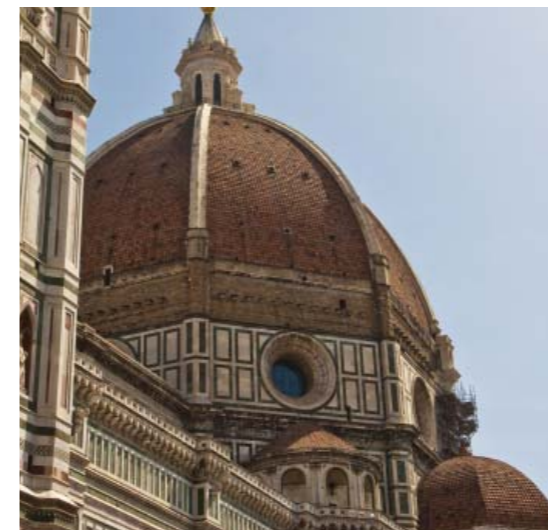
The Duomo (Florence Cathedral), Brunelleschi's masterpiece of structural design and engineering.
